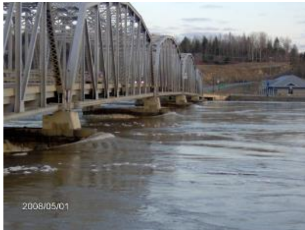
Perth-Andover Bridge at Spring Flood
