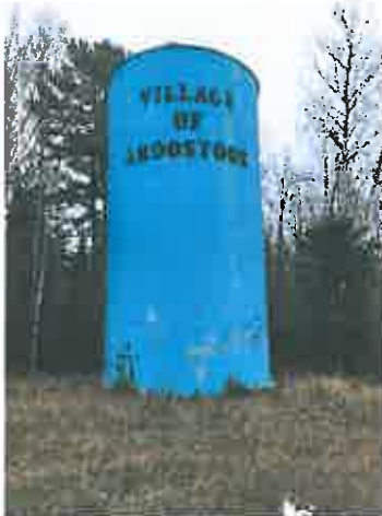
115,000 IG Steel Water Tank
