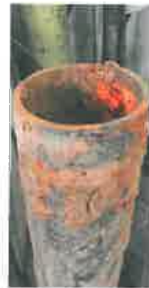
Water Pipe Section
