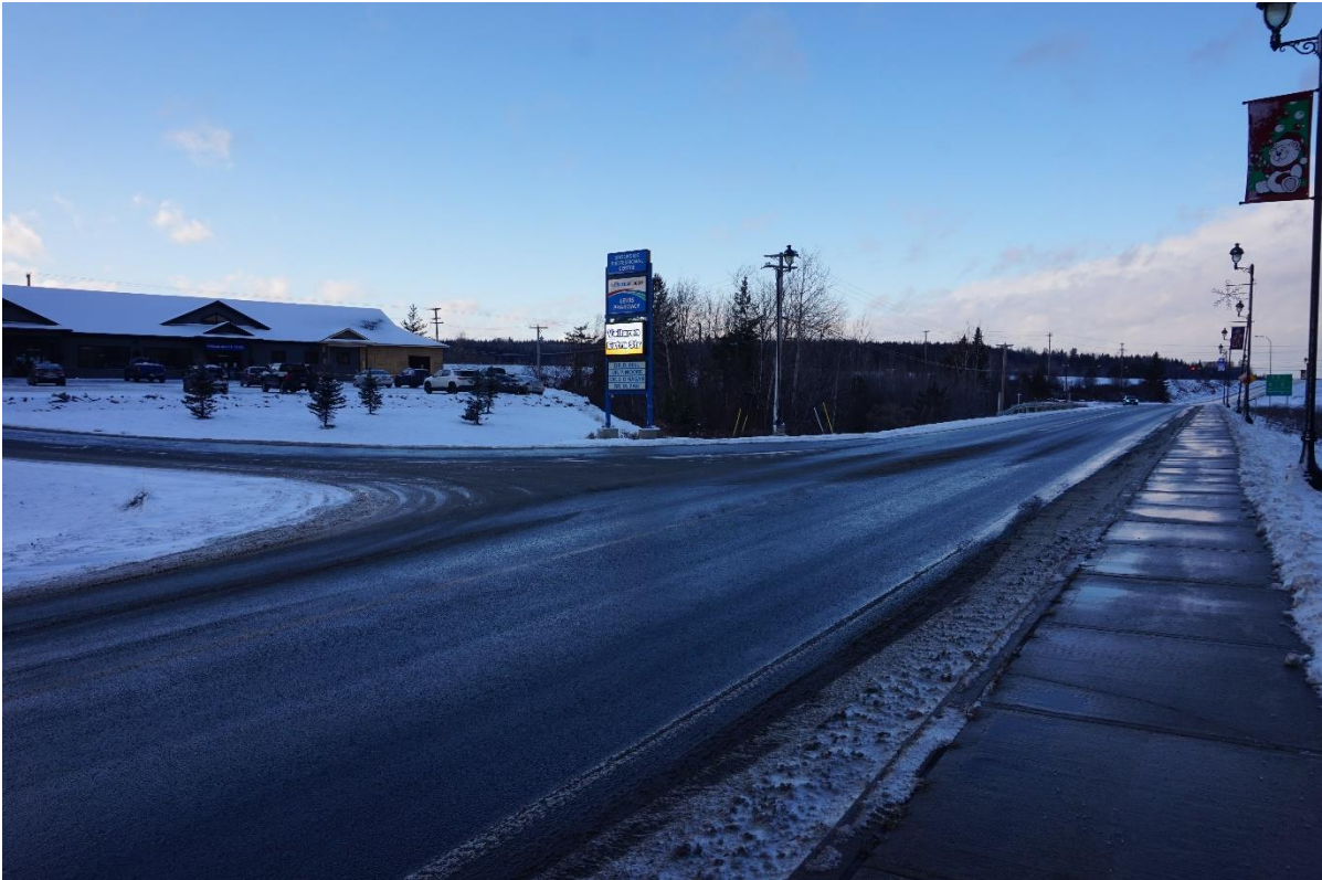
Figure 22: F. Tribe Road North Driveway - Northbound View
