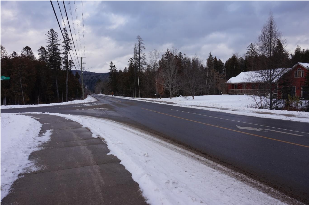
Figure 26: Fort Road @ Nissen Street - Eastbound View
