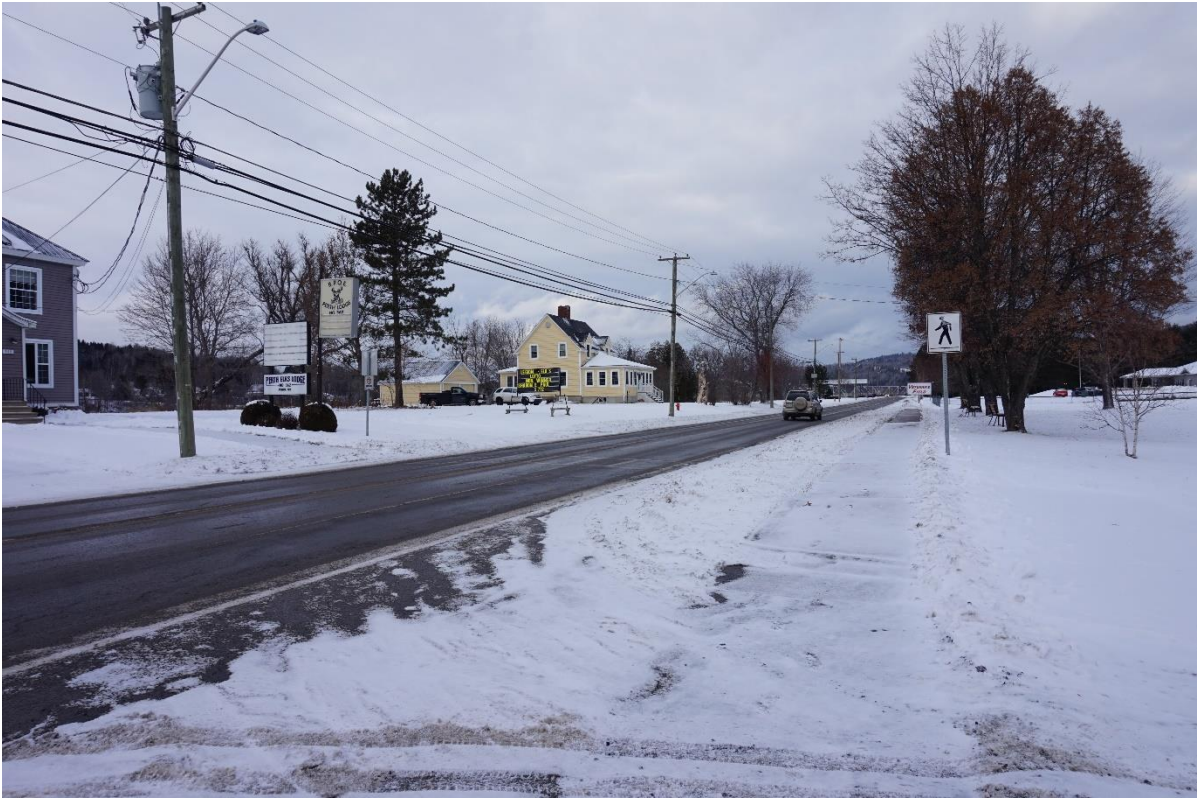
Figure 15: Elks Lodge Crosswalk - Northbound View
