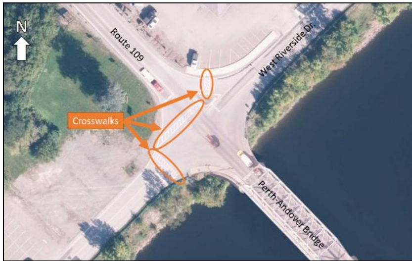
Figure 6: Bridge - Andover Crosswalk
