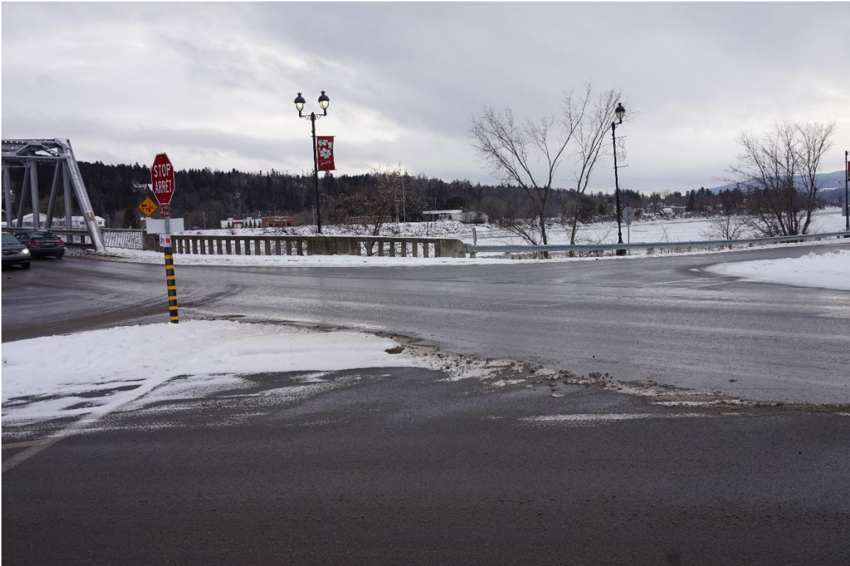
Figure 18: Bridge - Andover Crosswalk - Southeast View
