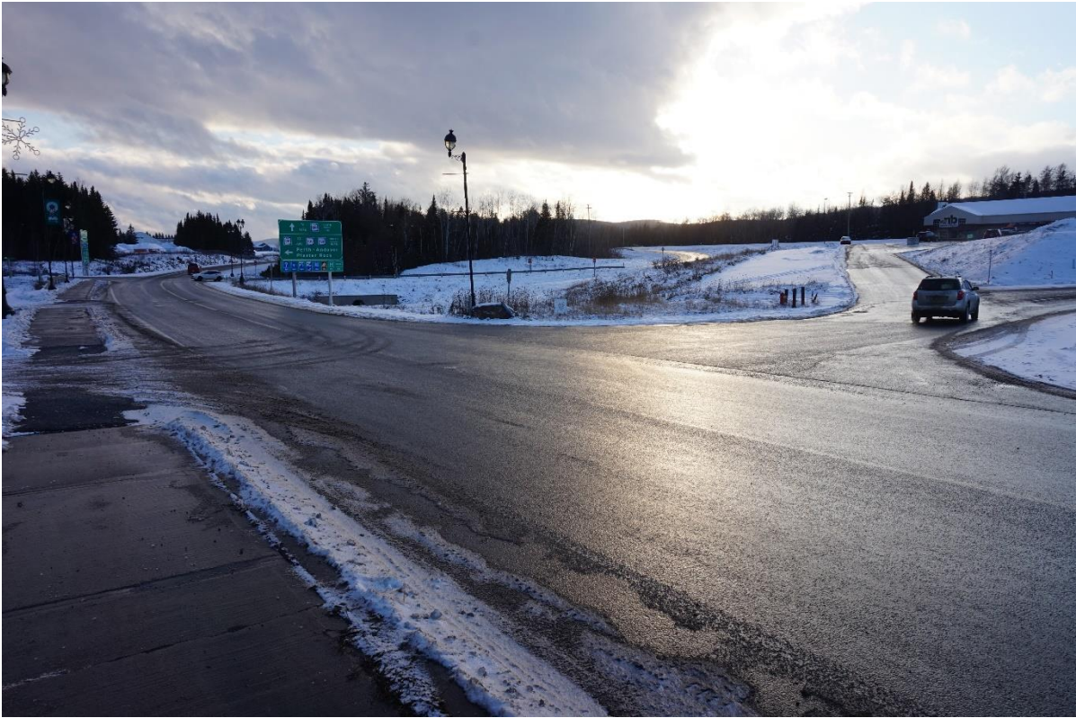
Figure 24: F. Tribe Road South Driveway - Southbound View
